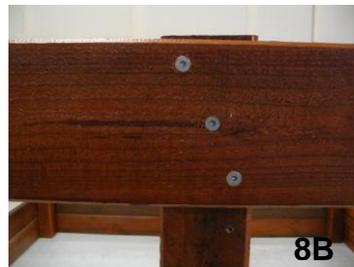
9. Cut any excess length off the posts such that they protrude 50mm to 60mm above the top of the frame.
